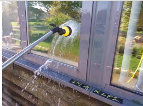
16. Window framework/joints/seals – spray tested – no result
