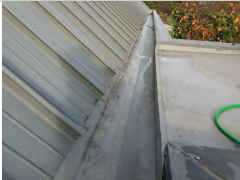
48. Single-ply waterproofed box gutter
