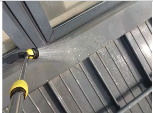
93. Flashing joints/base of windows - spray tested – no result
