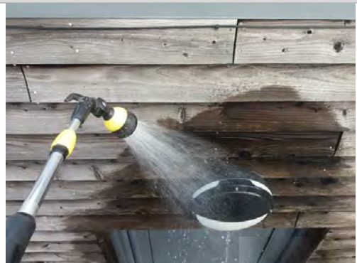
65. Light fitting – spray tested – no result
