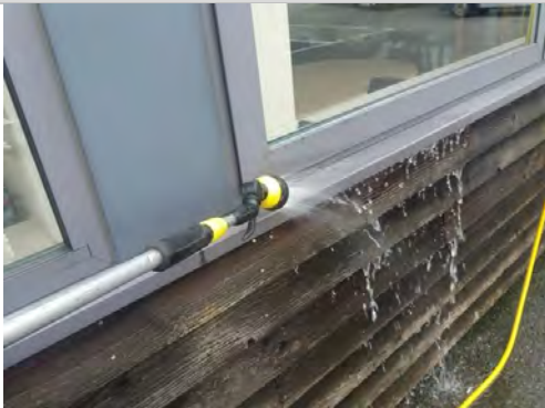
72. Window cills - spray tested – no result
