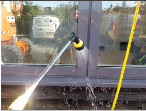
74. Window framework/joints/seals - spray tested – no result
