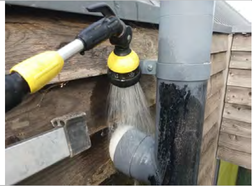
39. Penetration – spray tested – no result
