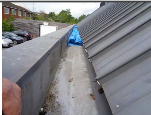
10 Tarpauline laid over gutter defects.
