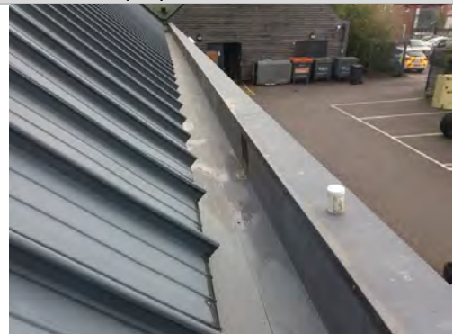
81. Visual inspection to box gutter waterproofing
