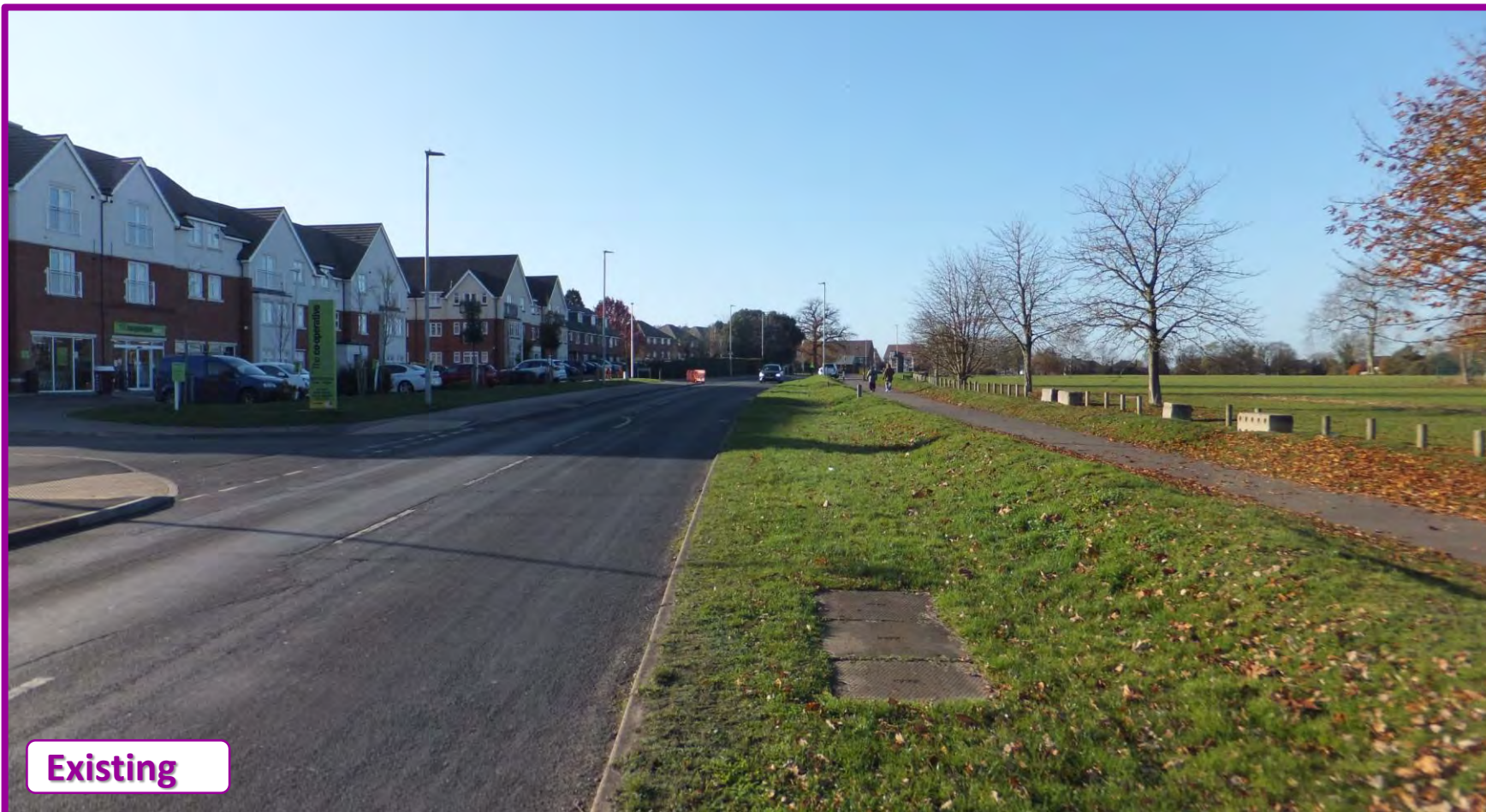
Image 2 – Woodlands Avenue / Louden Square Junction – Looking west
