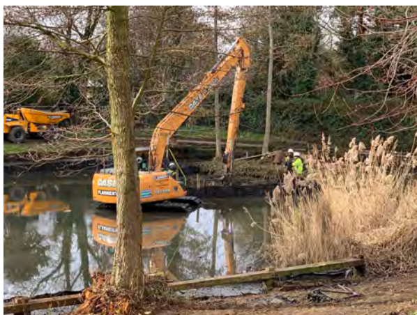
De-silting and boardwalk construction
